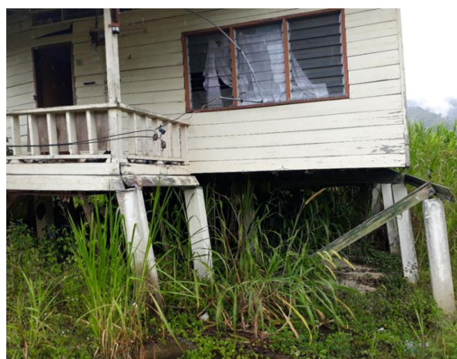
Figure 8: Extremely damaged on column structures caused by the seismic activities in the area.
