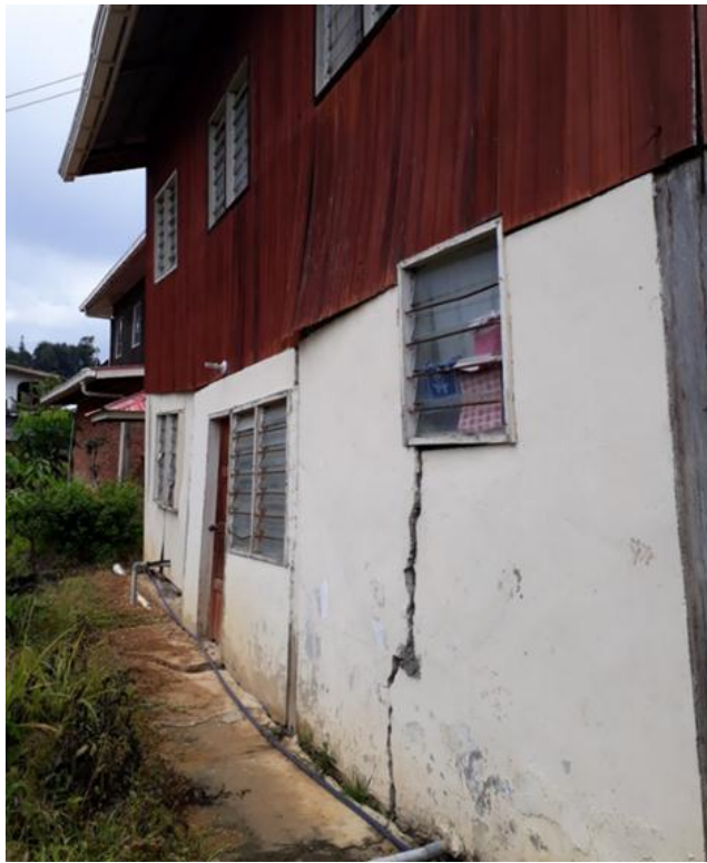
Figure 9: A house located in Kg. Lobou-Lobou Kundasang destroyed by the 2015 Ranau earthquake. The damage is very visible and dangerous, but the resident of the house is still living inside the house.
