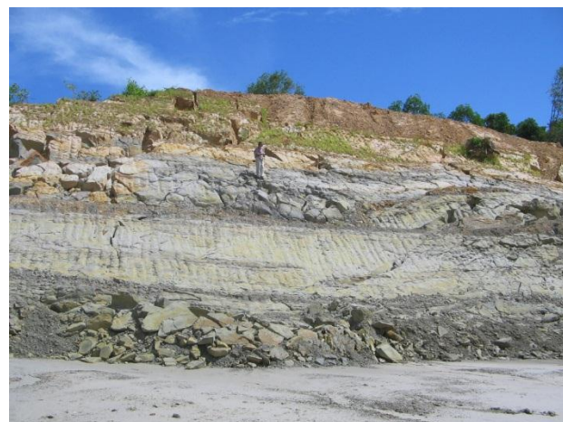
Figure 5: Outcrop generally consists of fine texture, cohesive materials, highly weathered to residual soil materials (Location: Sunny Estate)
