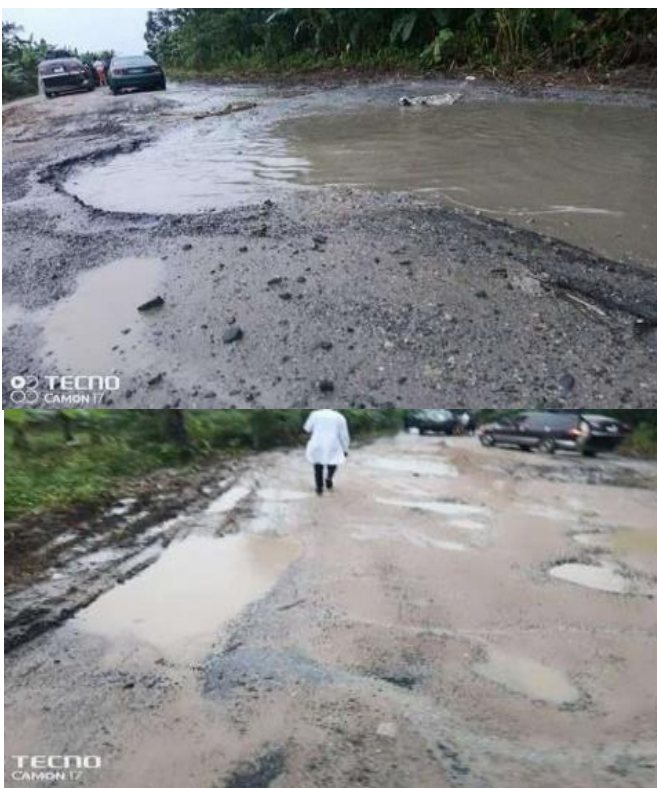
Plate 1: Specimen of a typical pothole on some of the Roads within the Study Area
