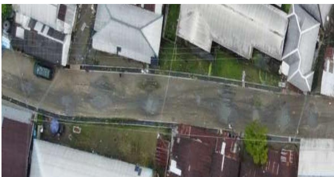
Figure 5: Orthophoto Map of the Section of Ebi's Mechanic Road in Yenagoa City
