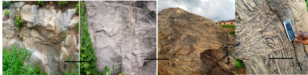
(b) Surface exposures and outcrops of migmatites and granite gneiss at different locations having being subjected to intense weathering, with noticeable fractures/fissures. In addition feldspathic and quartzo-feldspathic intrusion are also observed
