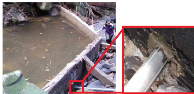
Figure 2: The spring-water catchment at the upper hill area, Bukit Bendera village and the plugged 5 inches PVC pipe.
