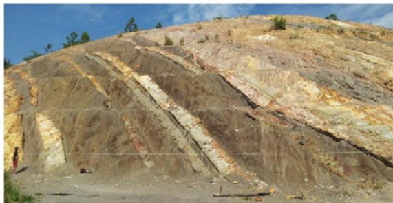
Photograph 3: Rock cut slope for slope A. Interlayer of thick shale and sandstone layers (Photograph orientation N 228°).
